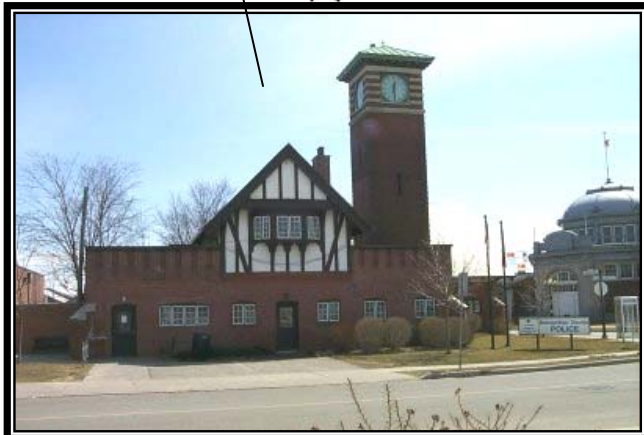
The Sub Station at Exhibition Place 275 Manitoba Dr. 416-808-1500
