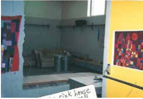
The first wall is opened up
