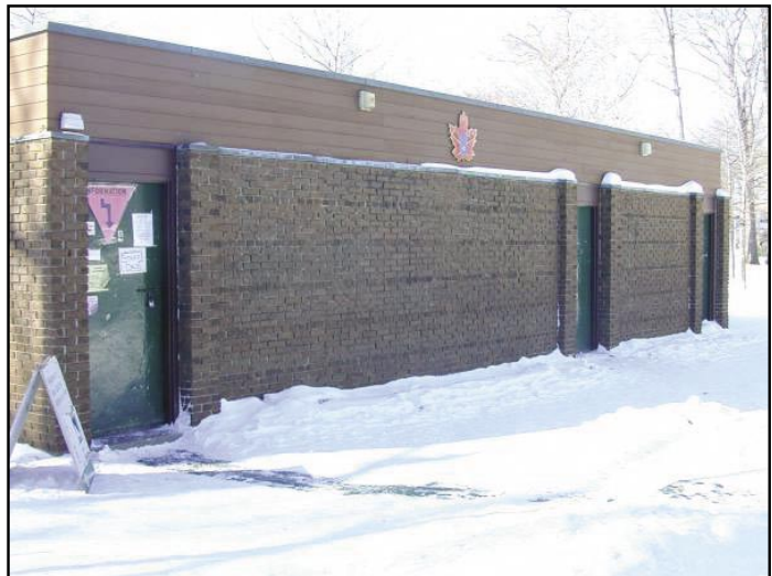
No windows in staff room, Kew Rink
